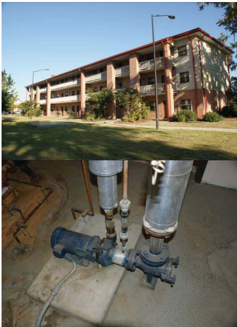
Barracks 1511 – 3HP Constant Speed End Suction Pump
