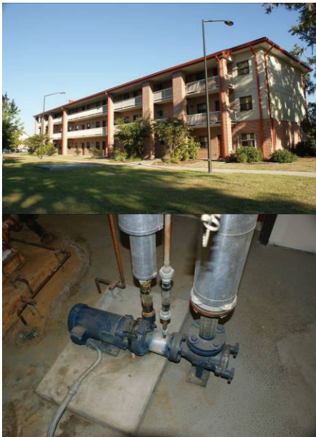
Barracks 1511 – 3HP Constant Speed End Suction Pump
